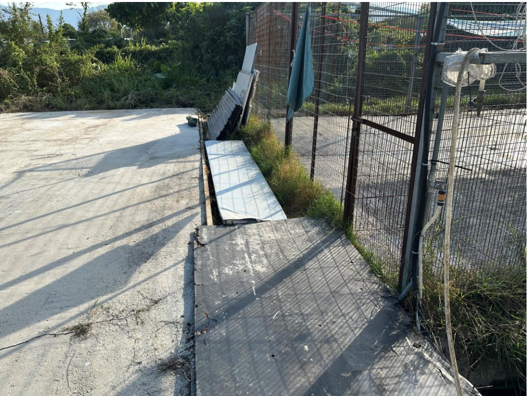
Photo 3: Drainage Network within Project Site
