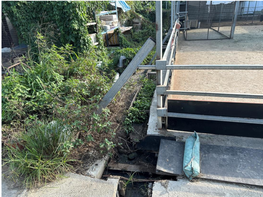
Photo 1: Drainage Network within Project Site
