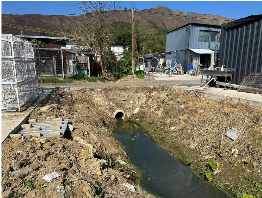
Photo 2: Natural Stream within Project Site
