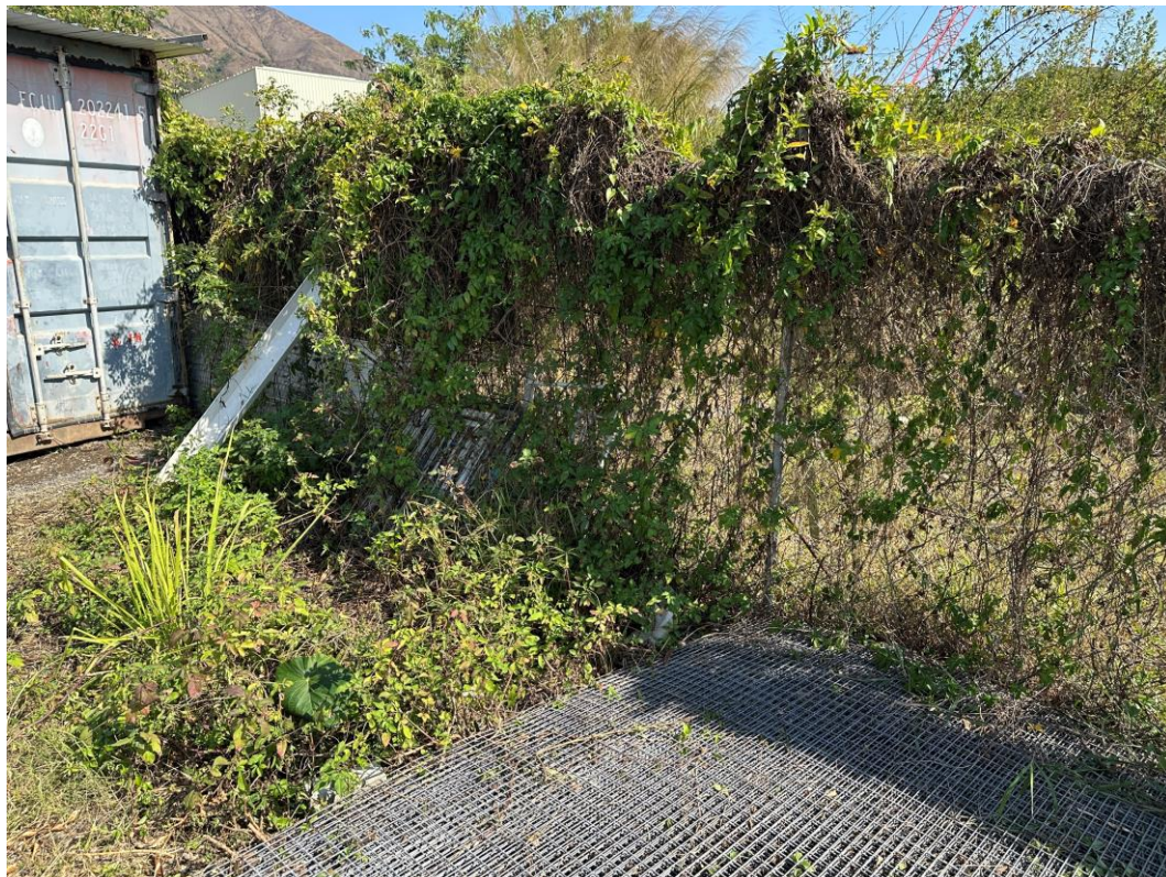
Photo 2: Hoarding without Concrete Footing
