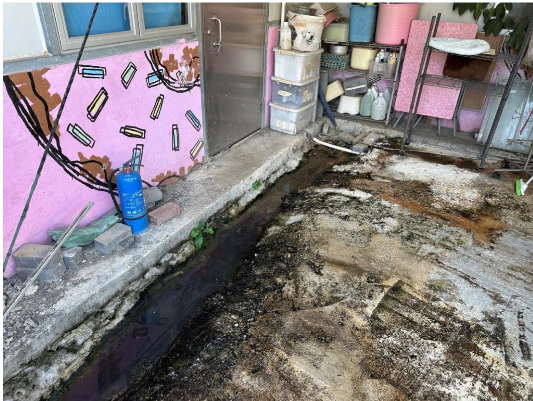
Photo 2: Drainage Network within Project Site
