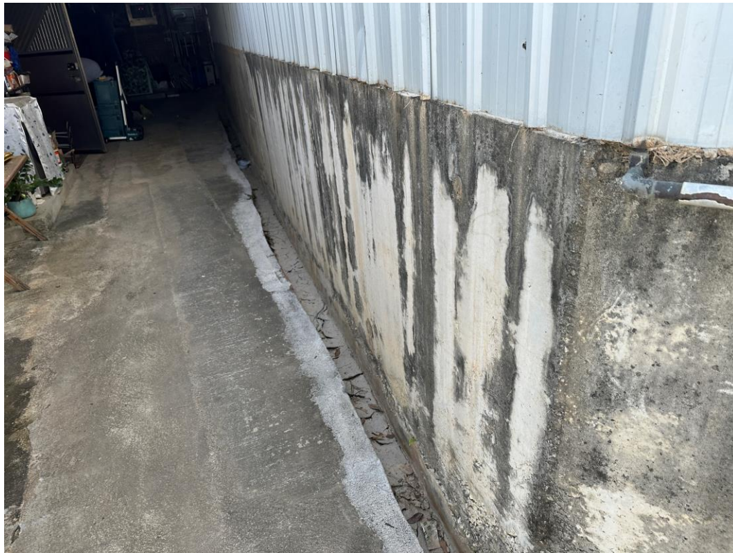
Photo 2: Concrete Footing at other premises
