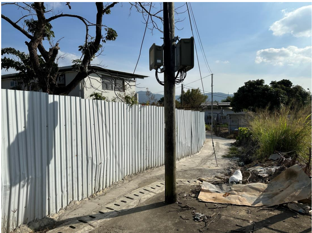
Photo 3: Hoarding with Concrete Footing
